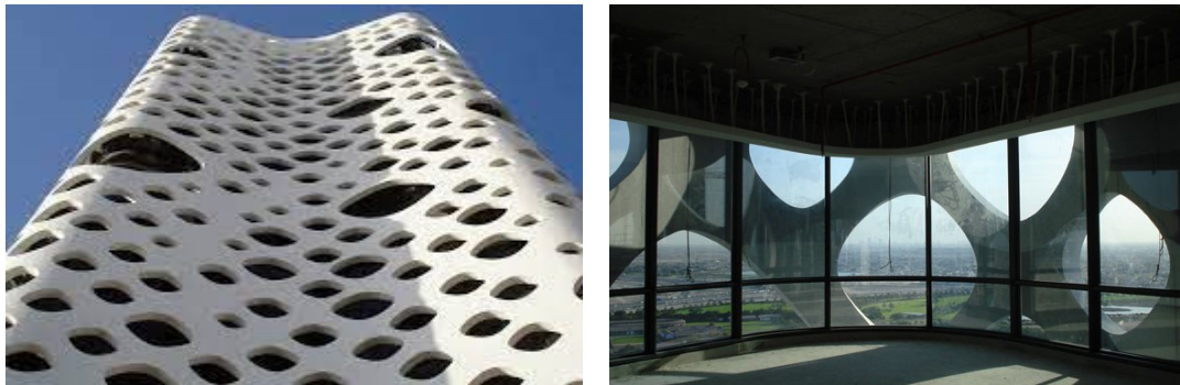
Figure 8. Façade perforations that act as solar screens - Al-Kodmany, 2014
