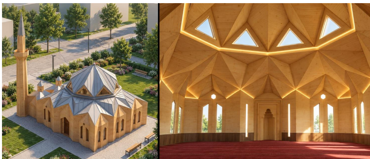
Figure 1. Architectural rendering illustrating the application of the Barkat timber folded plate system as a mosque, emphasizing its reinterpretation of historical Islamic architecture for a periodic use scenario.
