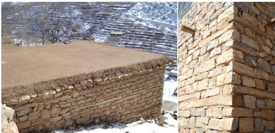
Figure 13. building construction components and materials in Tawela vernacular house, (photos: Authors)
