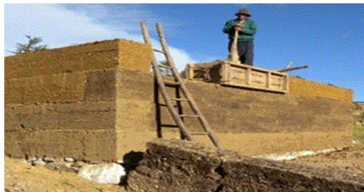
Rammed earth construction
